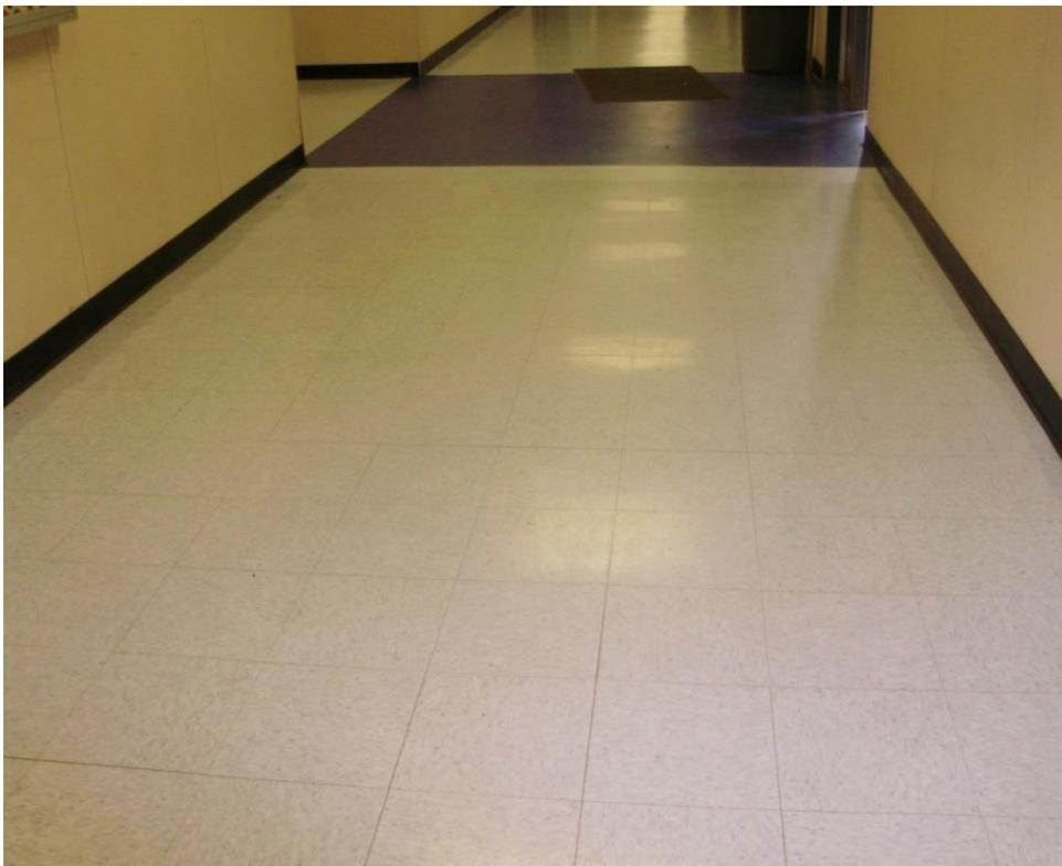
Figure 3-7. Polyurethane Coating at End of School Year
