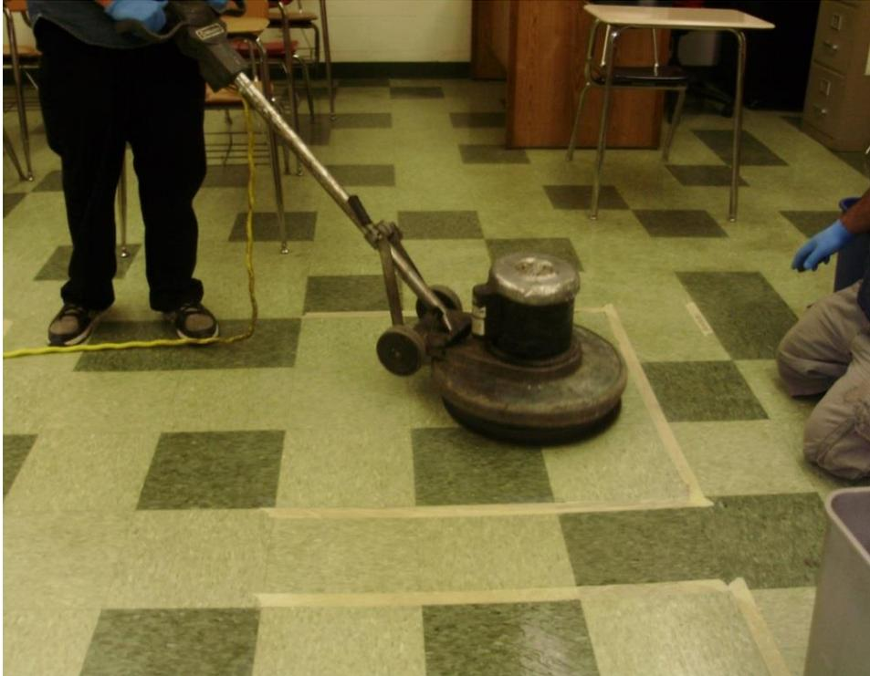
Figure 2-5. Floor Machine Stripping during Tests at Riverside USD
