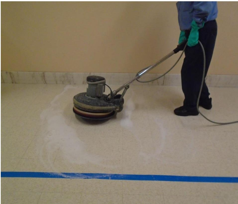
Figure 2-12. Using Floor Machine on Stripper during Testing at San Francisco City Hall
