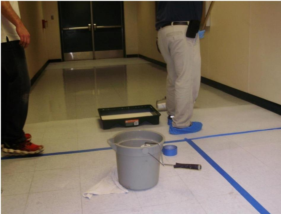
Figure 3-5. Workers Applying Polyurethane Coating
