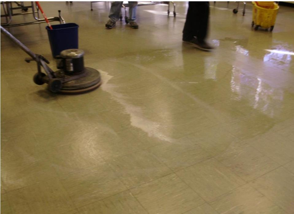
Figure 2-2. Floor Machine Stripping Wax
