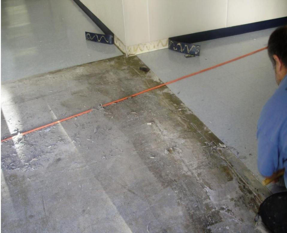
Figure 4-3. Workers Installing EcoPure Flooring
