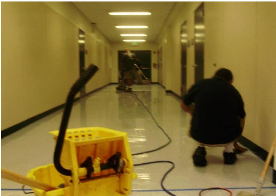
Figure 3-2. Workers Applying Vinyl Seal Coating
