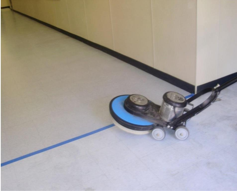
Figure 3-6. Hallway after Application of Polyurethane Coating
