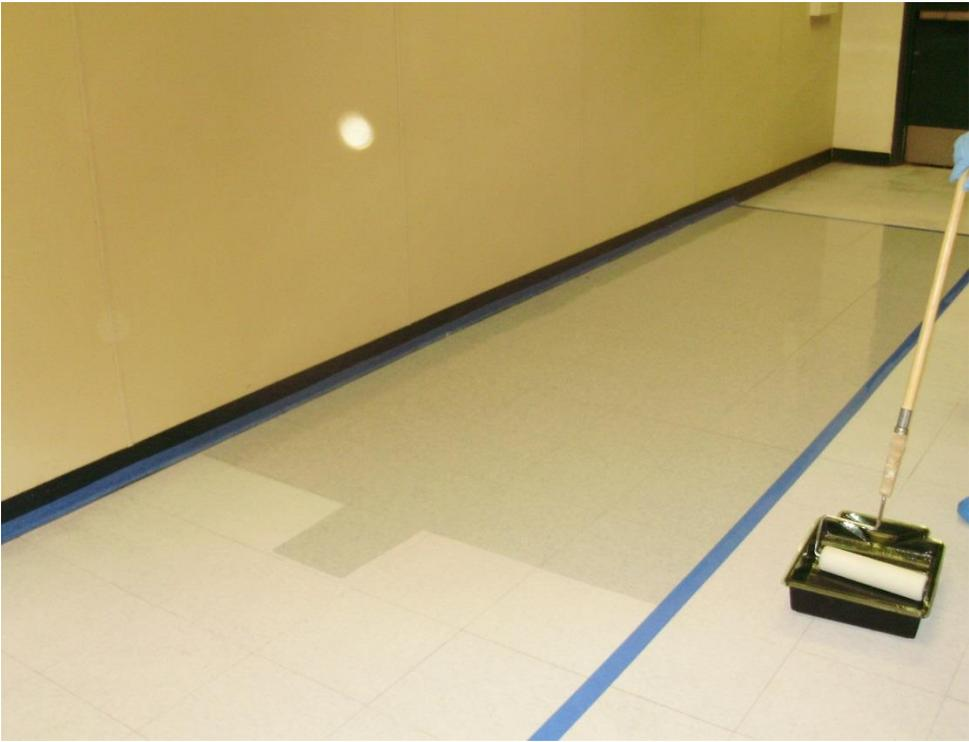
Figure 3-8. Workers Applying UV Coating
