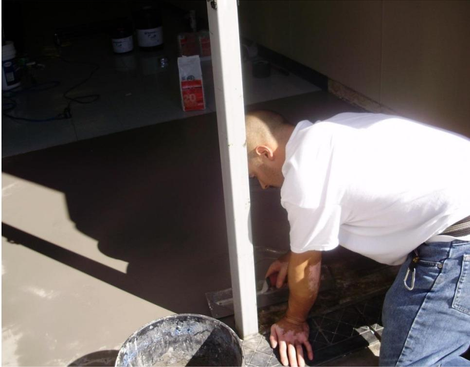
Figure 4-1. Workers Installing Optima IQ Flooring.
