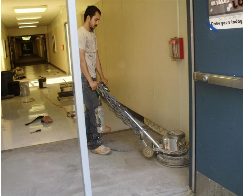
Figure 4-5. Workers Installing Omni Sports Flooring
