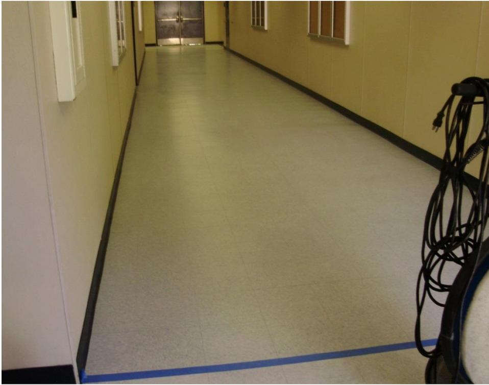
Figure 3-10. Hallway after Application of UV Coating
