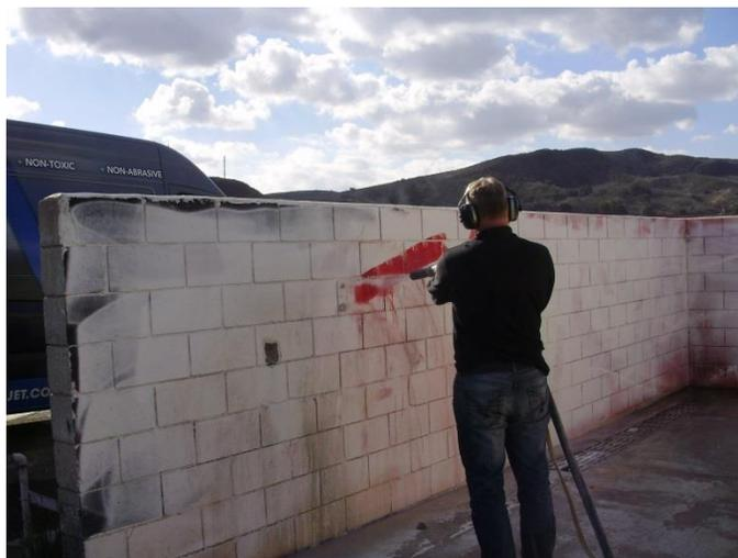
Figure 3-20. Glass blasting system removing paint from concrete wall
