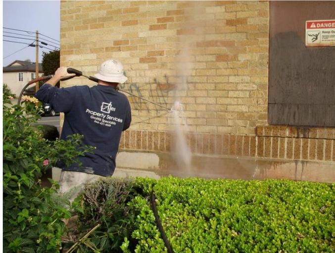
Figure 2-4. Contractor using soda blasting system
