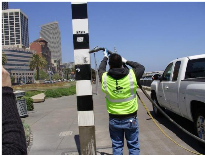
Figure 3-14. Glass blasting system removing graffiti from pole
