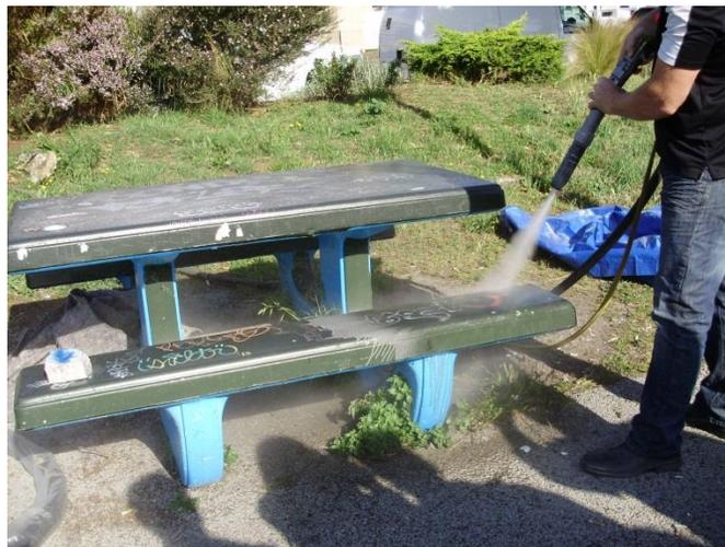
Figure 3-4. Blasting system removing graffiti from picnic table
