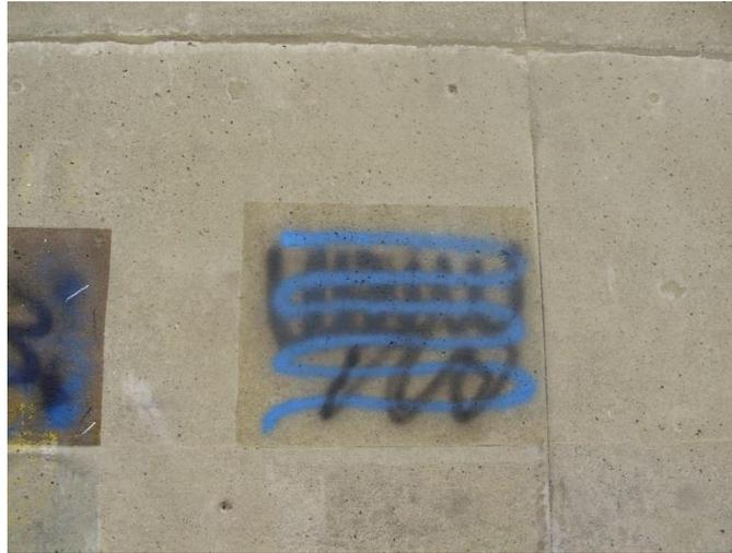
Figure 5-12. Coval coating on concrete wall with graffiti
