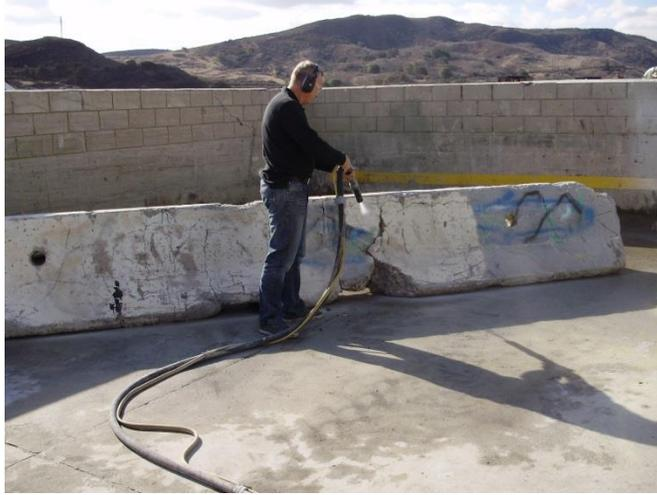
Figure 3-18. Dry ice blasting system removing paint from concrete barrier
