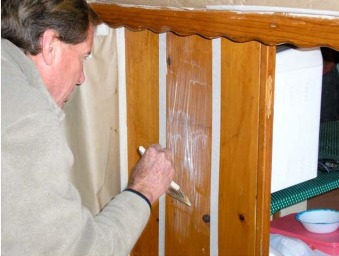
Figure 6-2. Brushing Stripper on Panel
