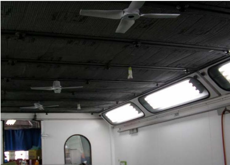
Figure 3-2. Three Ceiling Fan Drying System
