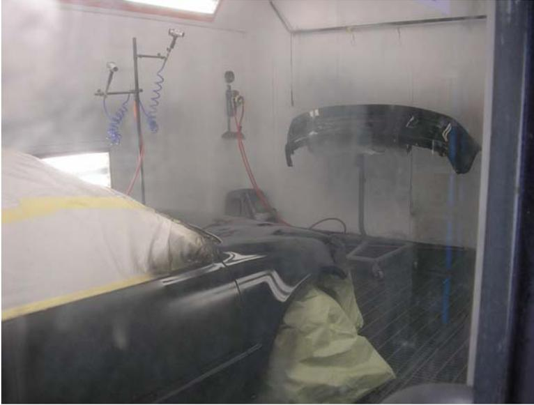
Figure 3-8. Car and Bumper Painted with Waterborne Base Coat at Autobody Shop #4
